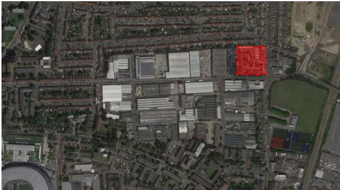
Image 3 - Aerial view of the site
