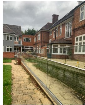
Rear of Kekewich House and linked extension building.
